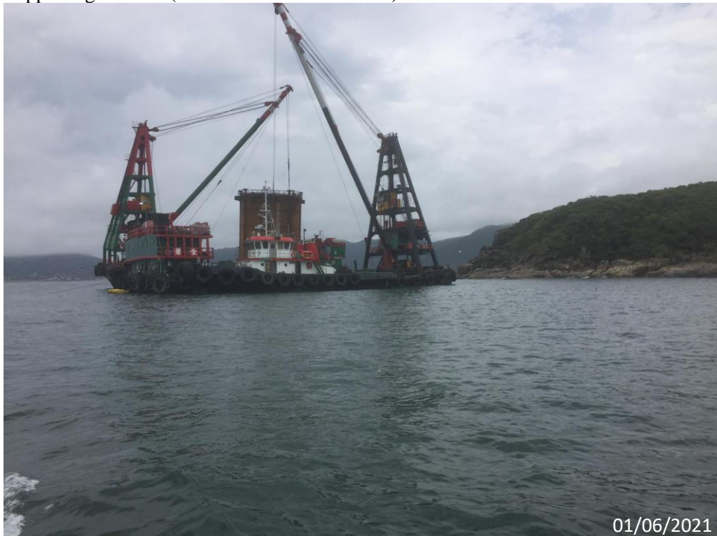
Supporting Photo 3 (Overview of Outfall Shaft)
