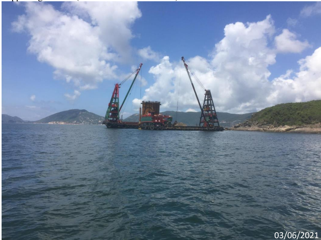
Supporting Photo 3 (Overview of Outfall Shaft)
