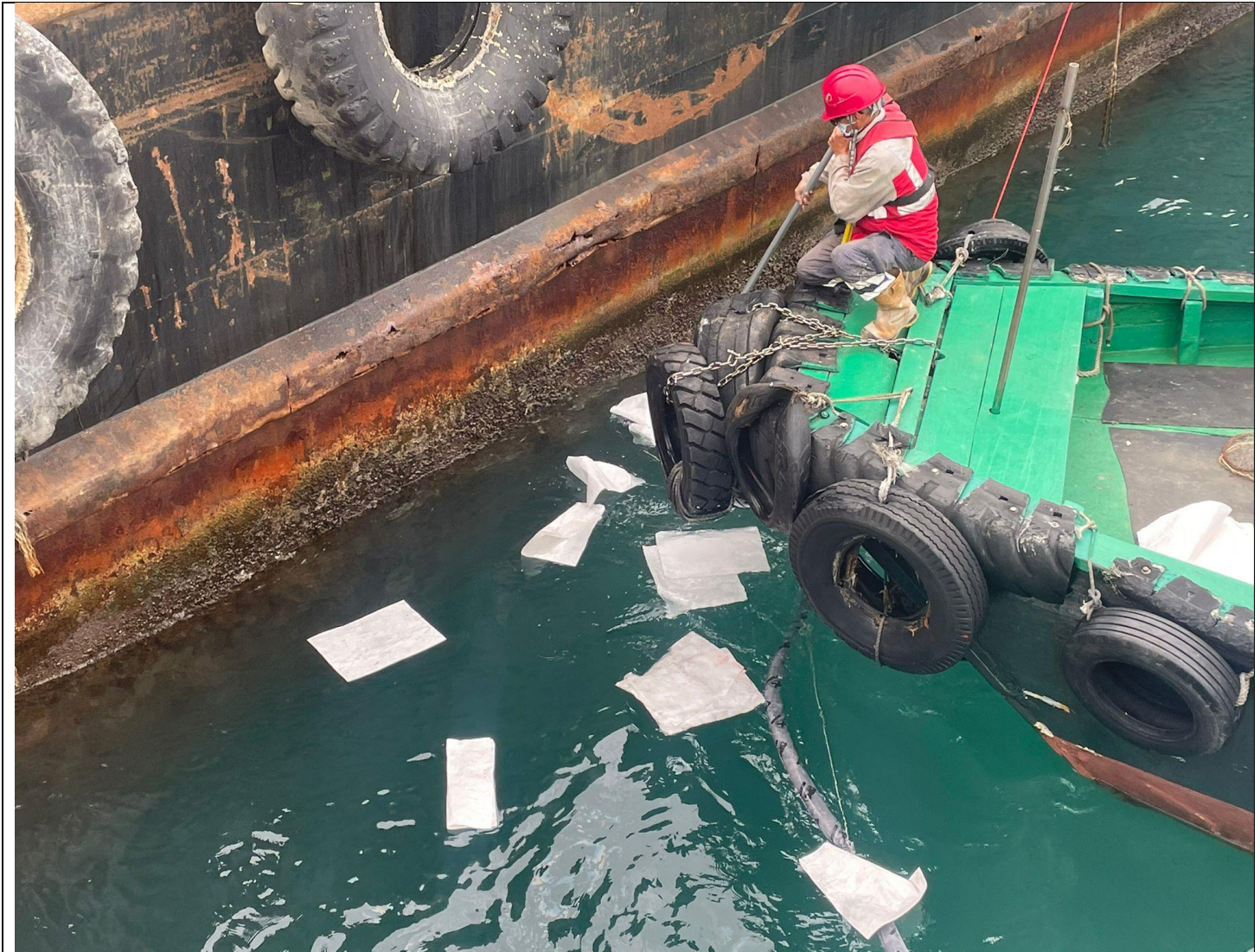
Figure 10: Emergency clean up measures on any residue oil spillage
