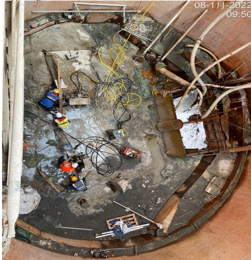
Supporting Photo 12 (Overview from inside the caisson at WSR37)
