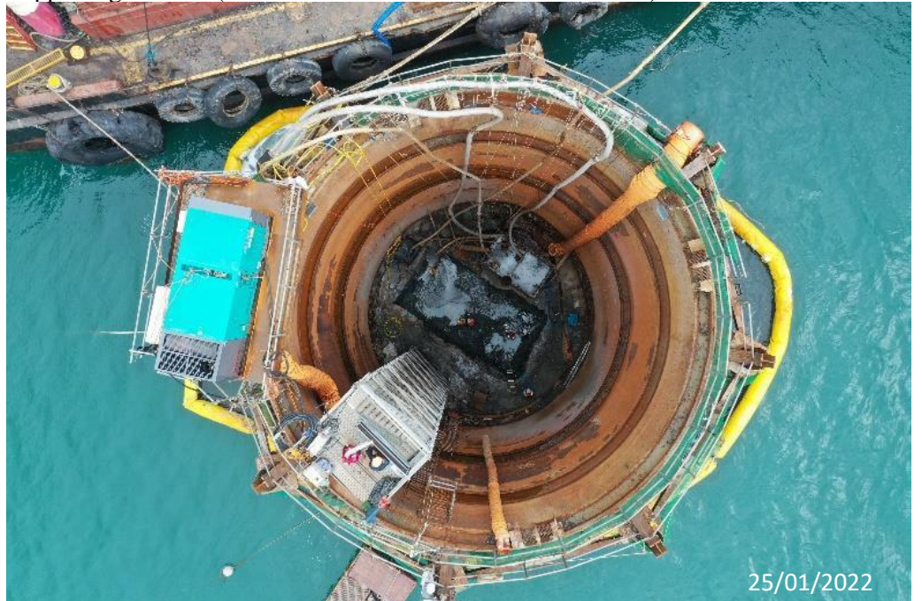
Supporting Photo 6 (Caisson Conditions at Outfall Shaft Area)
