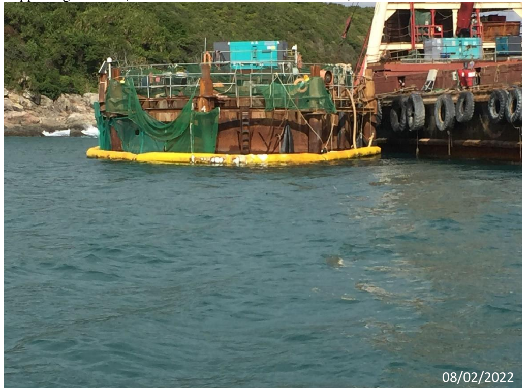
Supporting Photo 8 (Sea Conditions at Outfall Shaft Area)
