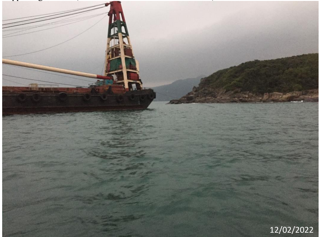
Supporting Photo 4 (Sea Conditions at Outfall Shaft Area)
