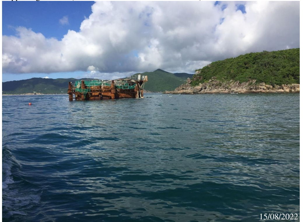
Supporting Photo 6 (Sea Conditions at Outfall Shaft Area)
