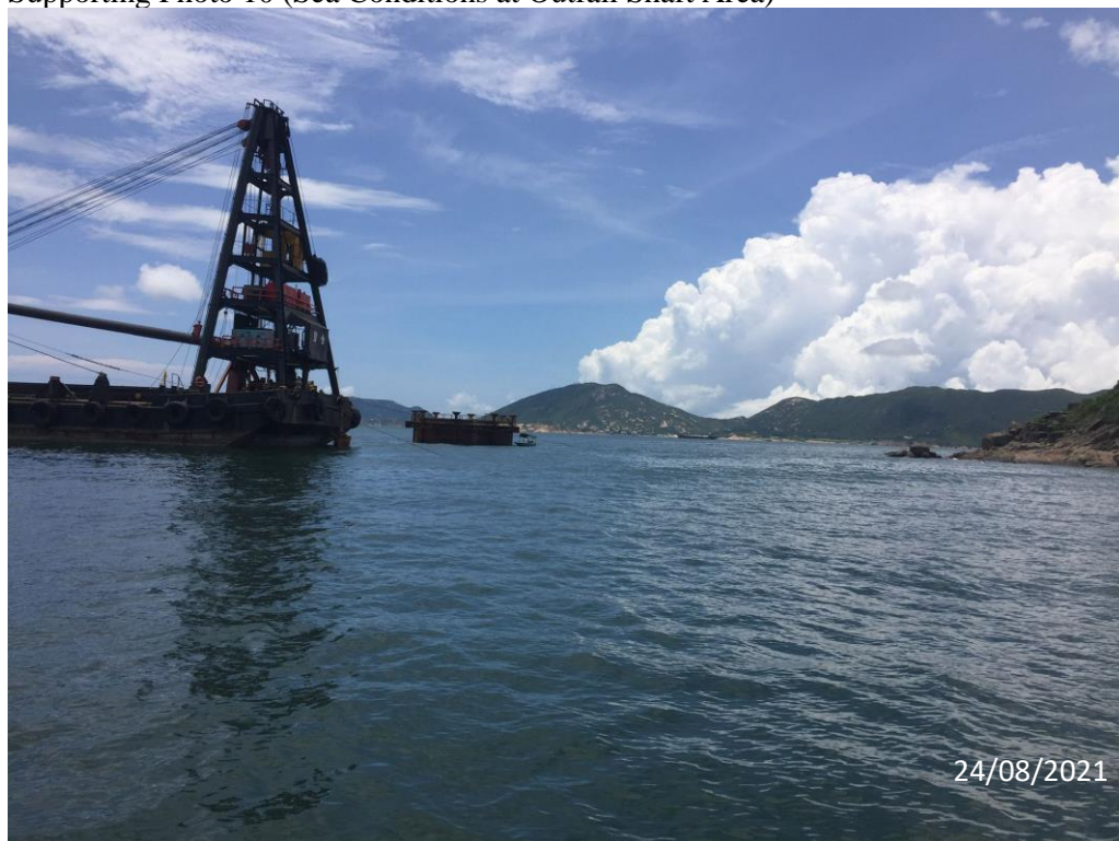
Supporting Photo 10 (Sea Conditions at Outfall Shaft Area)
