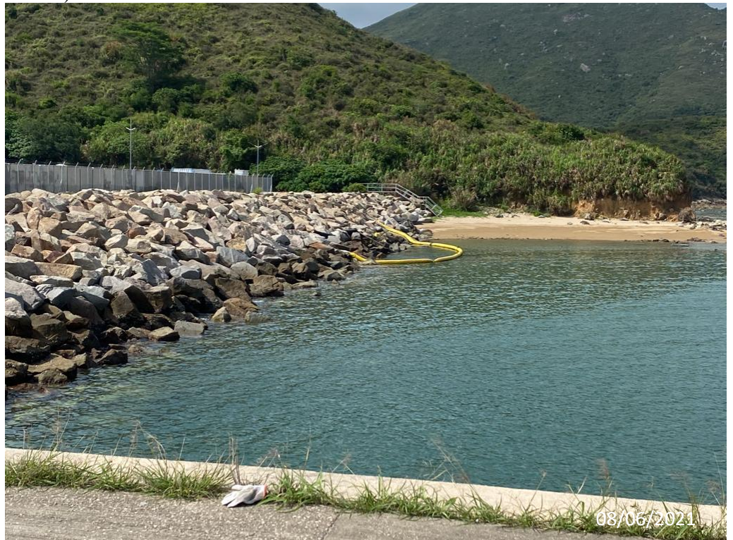
Supporting Photo 13 (Conditions of the Protective Silt Curtain at the Inland Water Outfall)
