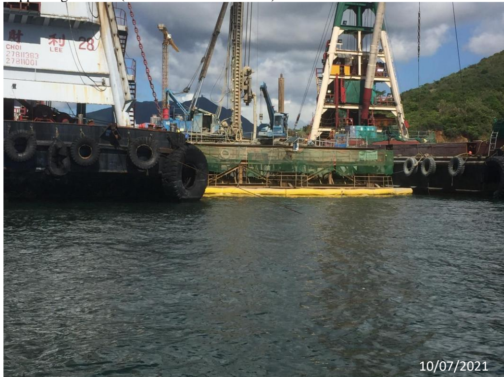
Supporting Photo 3 (Overview of Intake Shaft)
