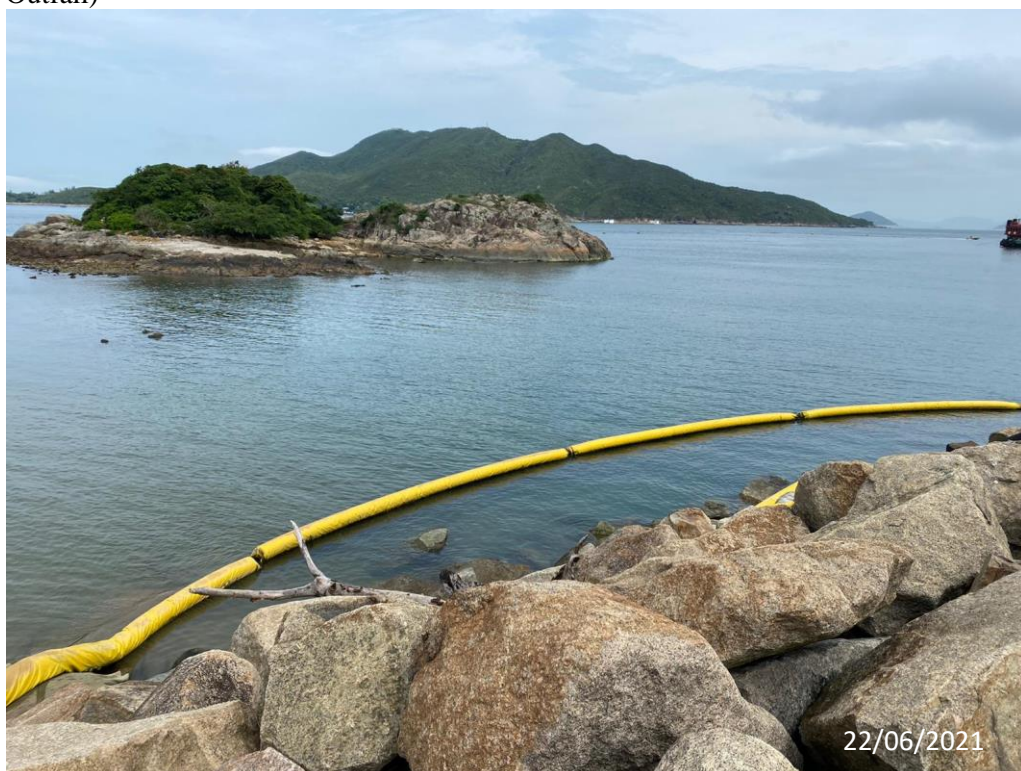
Supporting Photo 6 (Conditions of the Protective Silt Curtain at the Inland Water Outfall)
