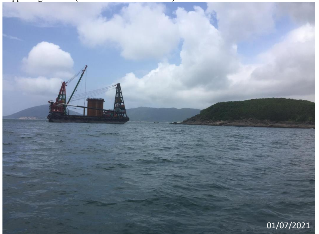
Supporting Photo 3 (Overview of Outfall Shaft)
