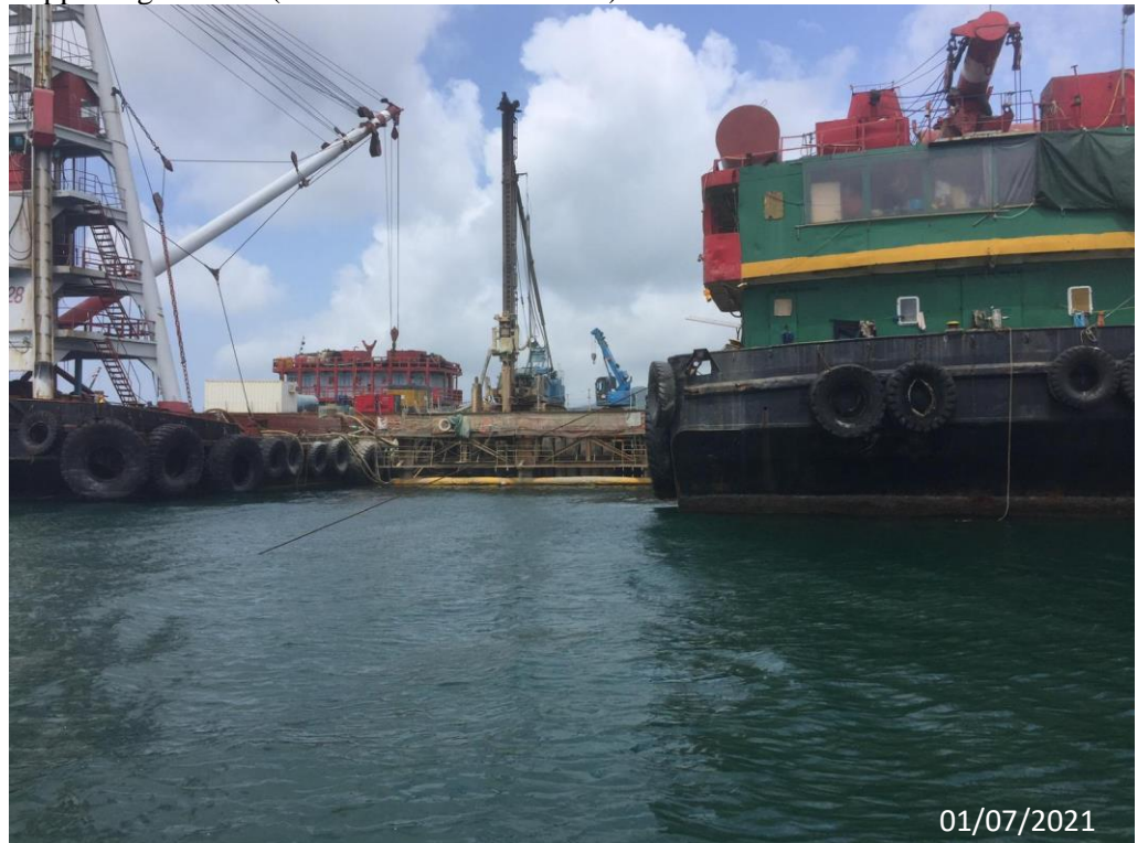
Supporting Photo 2 (Overview of Intake Shaft)
