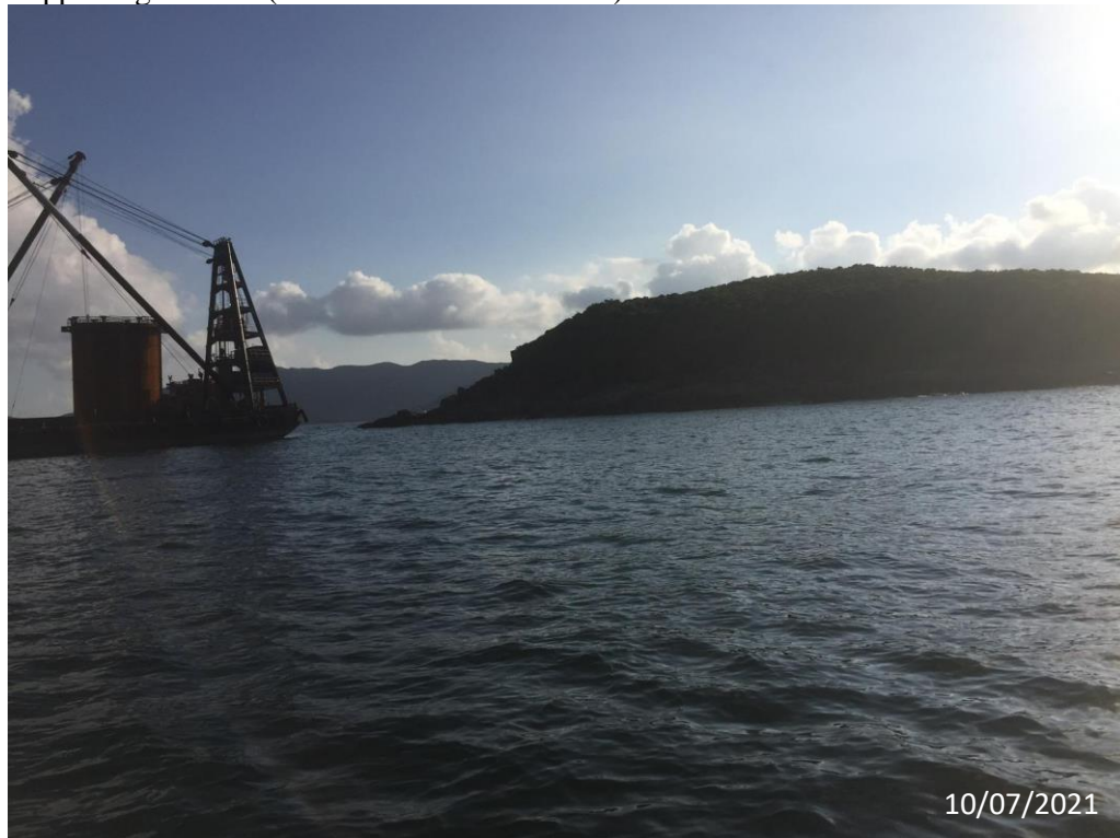
Supporting Photo 4 (Overview of Outfall Shaft)
