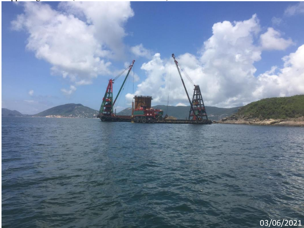
Supporting Photo 3 (Overview of Outfall Shaft)
