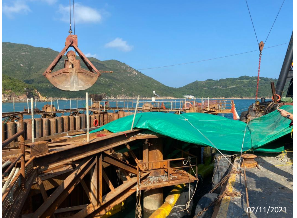
Supporting Photo 7 (Mitigation Measures during Trial Dredging on 02/11/2021)
