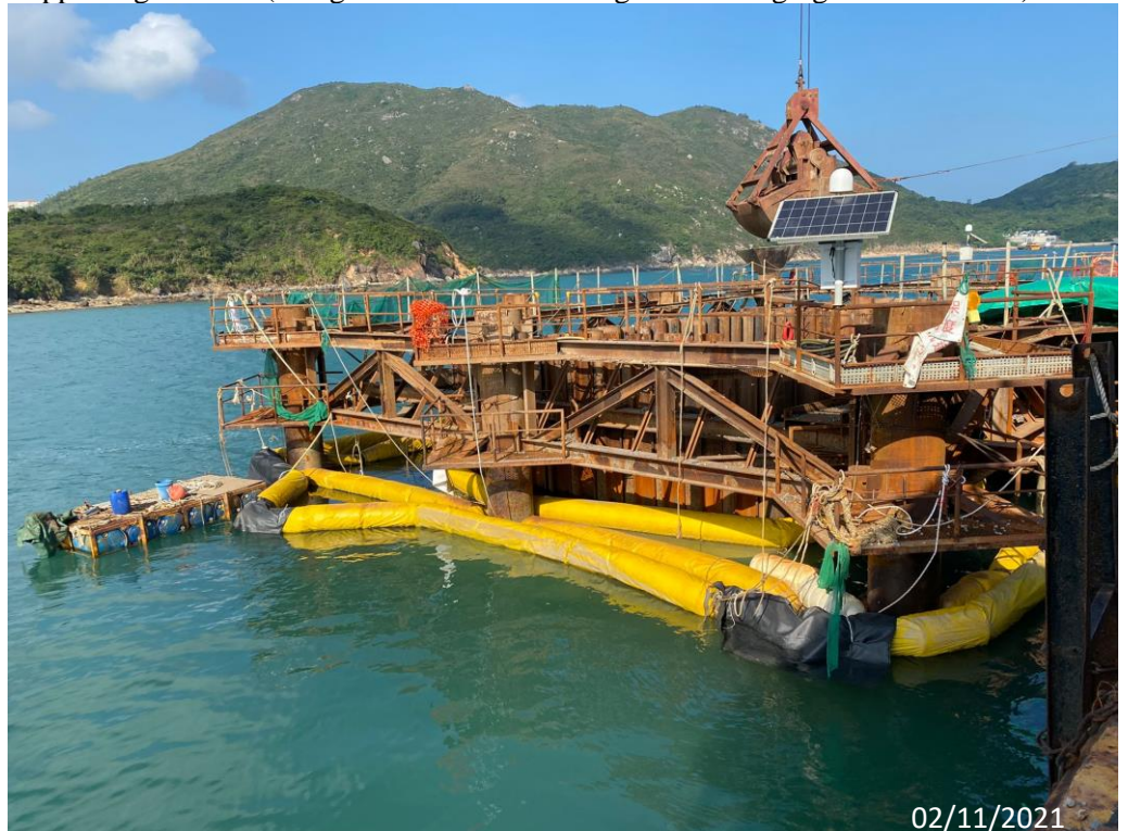
Supporting Photo 6 (Mitigation Measures during Trial Dredging on 02/11/2021)
