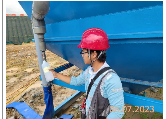
By main contractor at KNP site
