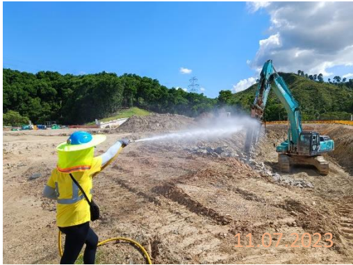
By subcontractor at KNP site
