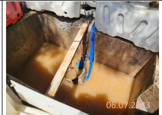
By main contractor at KNP site
