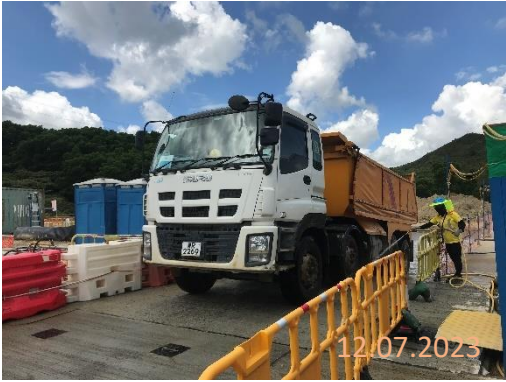
By main contractor at KNP site
