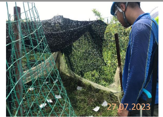
By subcontractor at KNP site
