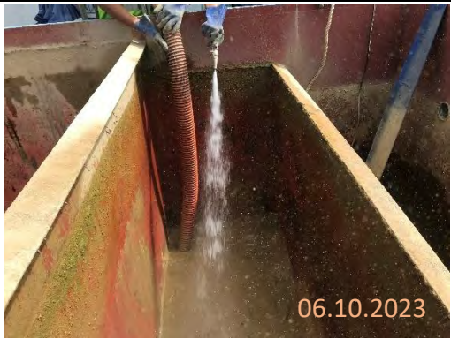
By main contractor at KNP site
