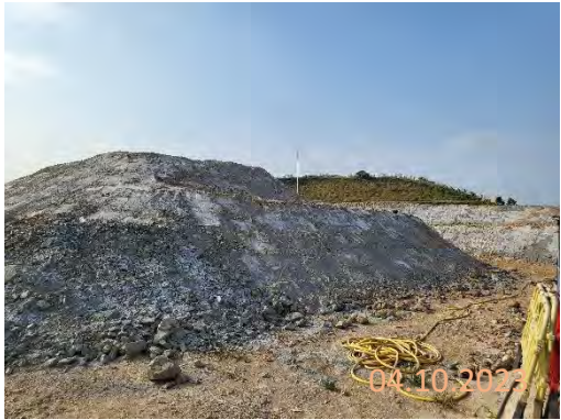
By main contractor at KNP site
