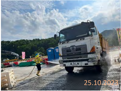
By main contractor at KNP site
