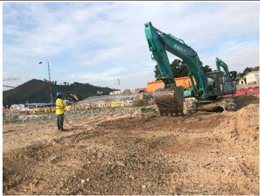
By main contractor at KNP site
