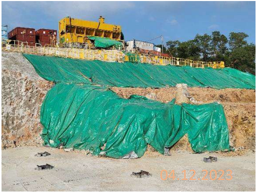
By main contractor at KNP site
