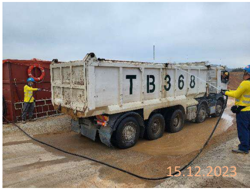
By main contractor at KNP site
