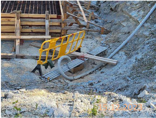
By main contractor at KNP site
