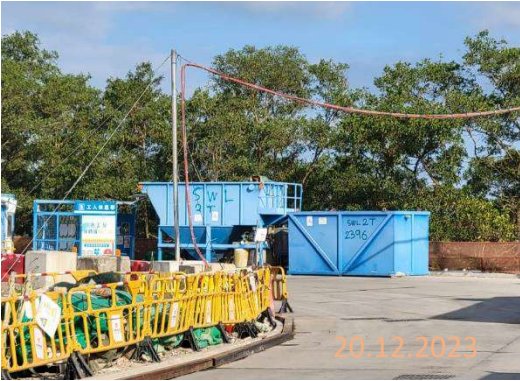
By main contractor at KNP site
