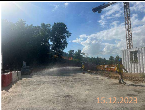
By subcontractor at KNP site
