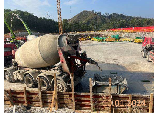
By subcontractor at KNP site
