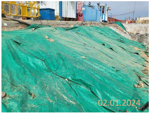
By main contractor at KNP site
