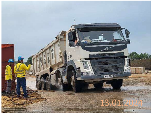
By main contractor at KNP site
