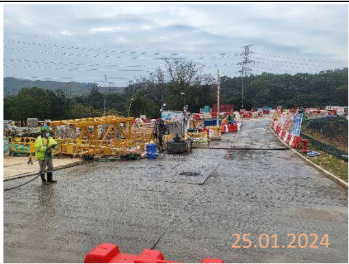
By subcontractor at KNP site
