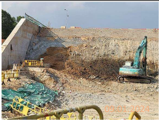
By main contractor at KNP site
