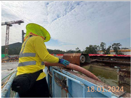
By main contractor at KNP site
