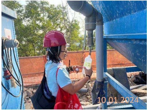
By main contractor at KNP site
