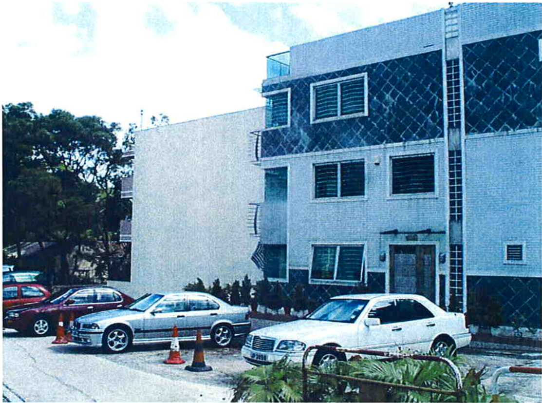
Monitoring Point CNM 1 – Wu Kwai Sha New Village
