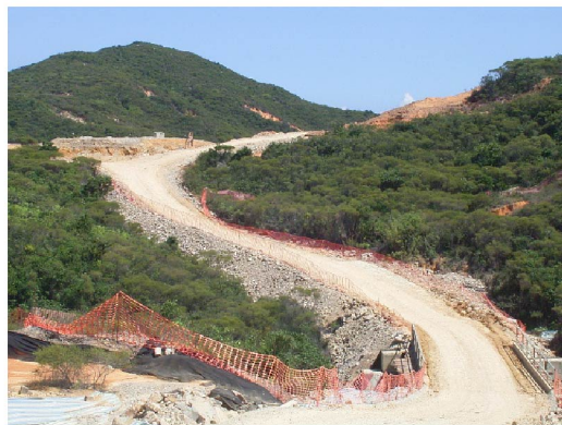
The haul road beyond Stream A
