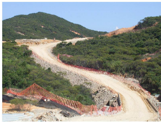
The haul road beyond Stream A
