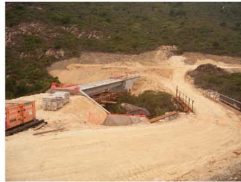
Temporary bridge and permanent bridge at Stream C
