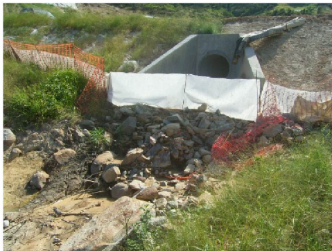
New drain near Stream B2
