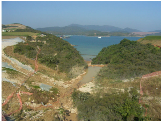
Stream A and the temp bridge area to be restored
