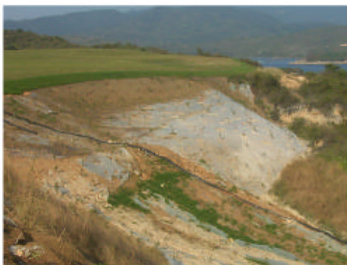
Stream A channel restored by planting & hydroseeding
