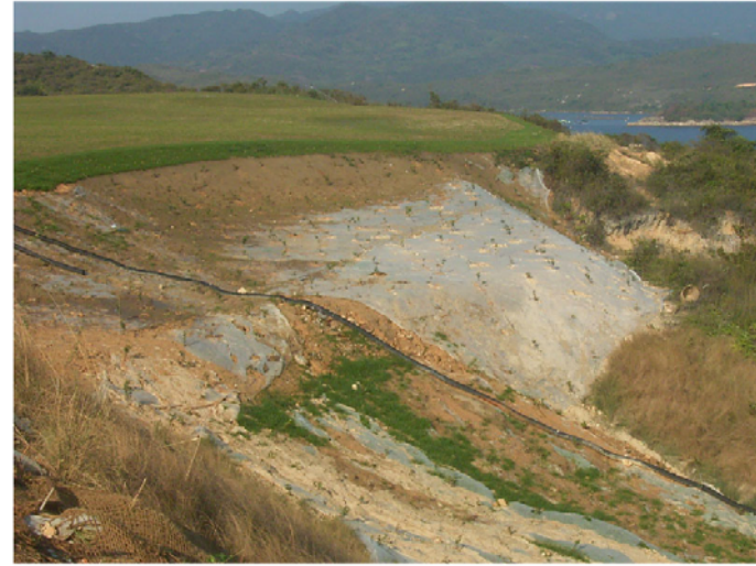
Stream A channel restored by planting & hydroseeding
