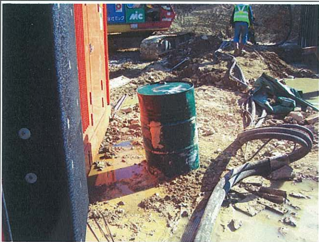
2.) The diesel drum was placed bare ground without drip tray.
