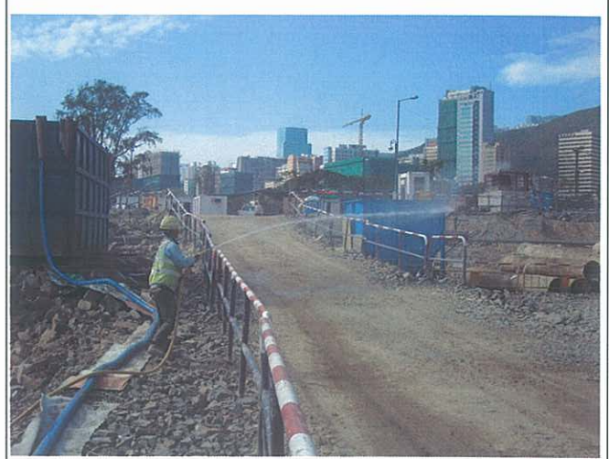
1.) Watering was carried out at the haul road.
