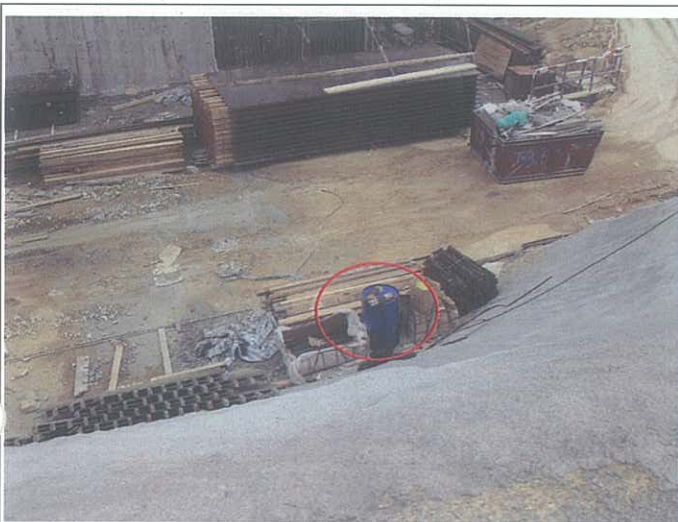
2.) Chemical drum without drip tray was observed at EP.
