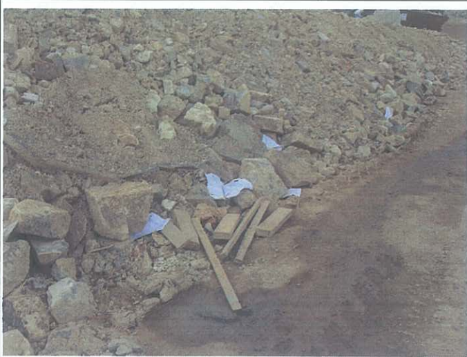
2.) General refuse was observed at fill material of stockpile.
