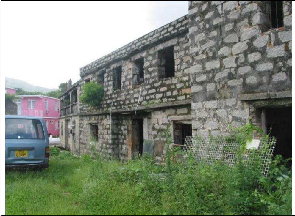
Photo 17: No 10 - Large house
