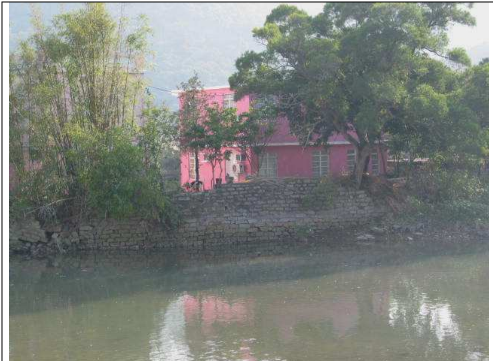
Photo 2: No 2 - Retaining – riverside wall
