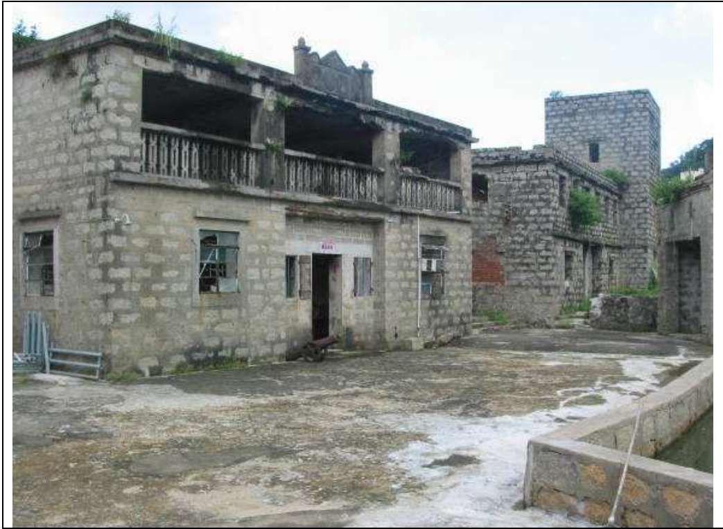
Photo 3: No 3 - Large Central House of "Yu Tak Li Wai" – Front view
