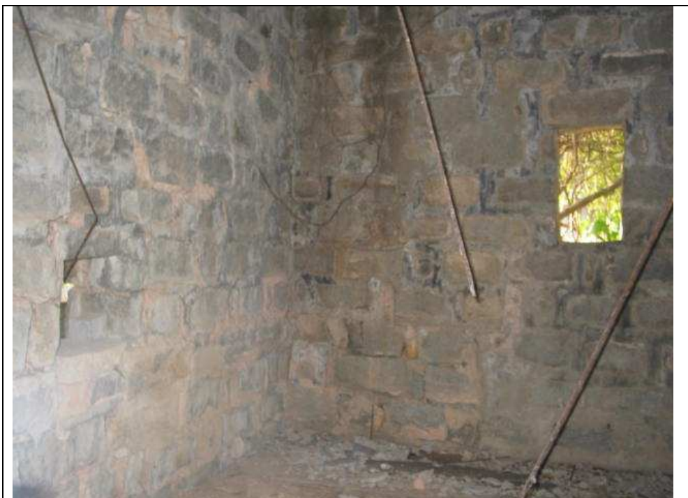
Photo 16: No 9 – Latrine (interior)
