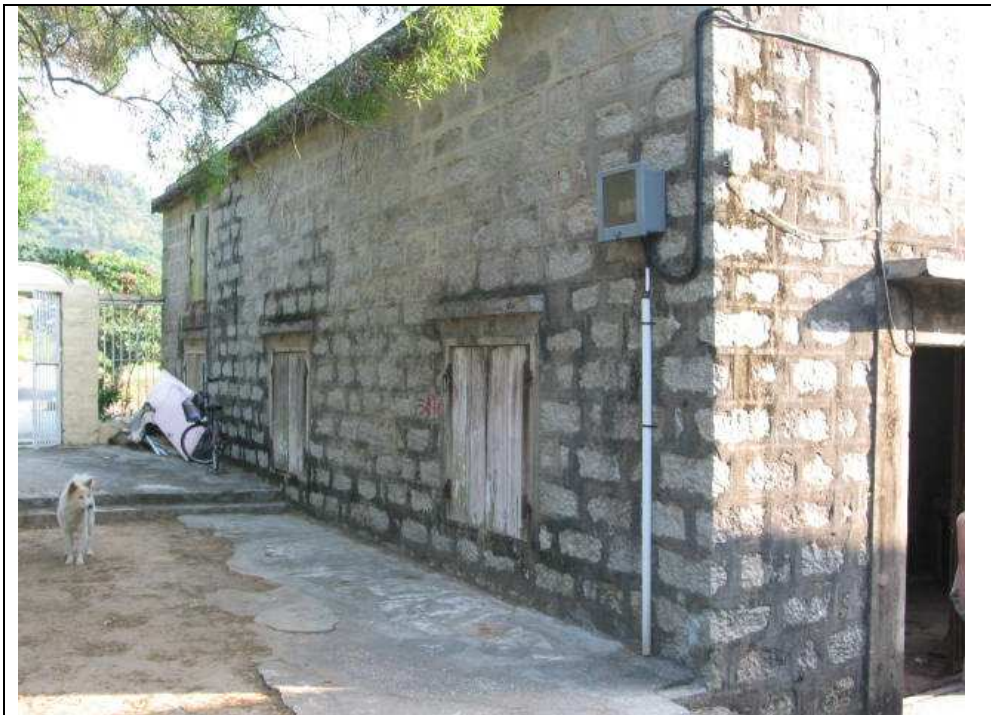
Photo 18: No 10 - Large house (Rear wall)
