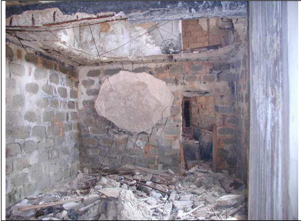
Photo 19: No 10 - Large house (Interior)
