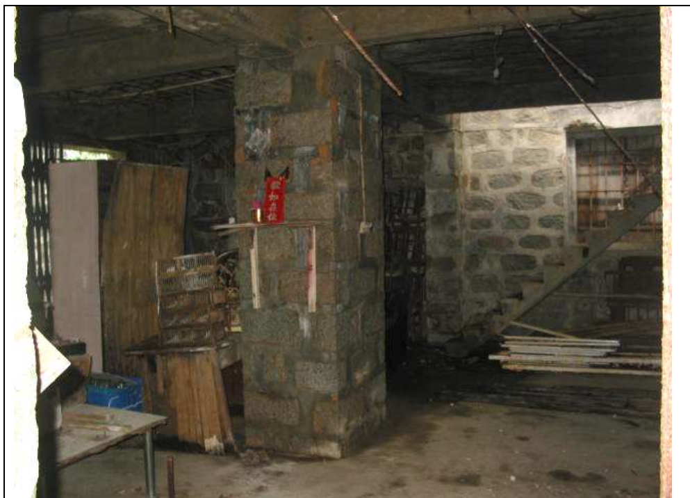
Photo 20: No 10 - Large house (larger main room)
