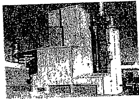
SO 2 sorption for exhaust gas from a tunnel kiln for bricks
