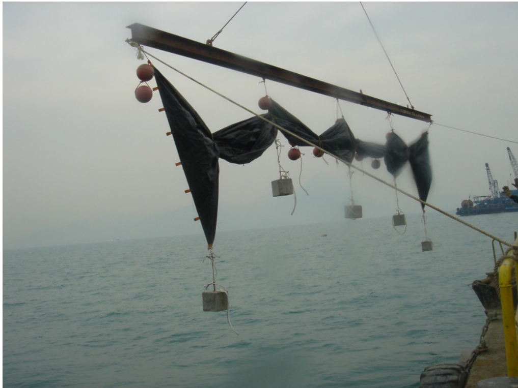
Photo 1 Preparation Works on the Work Barge.
