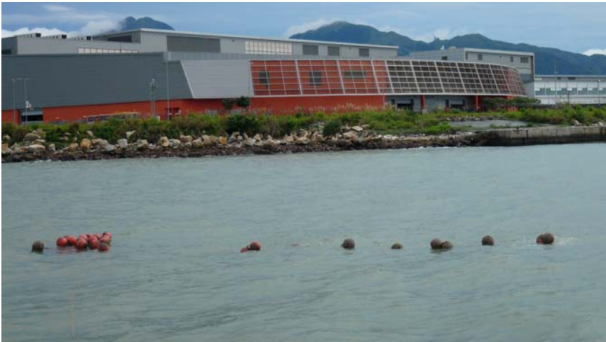
A.R. silt curtain being floated on the surface
