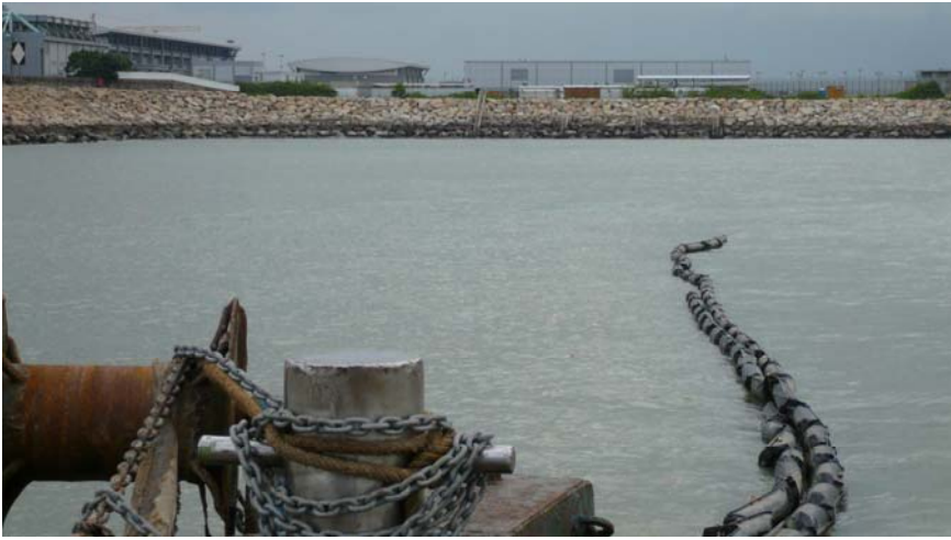
Recovering of Curtain from Water Intake
