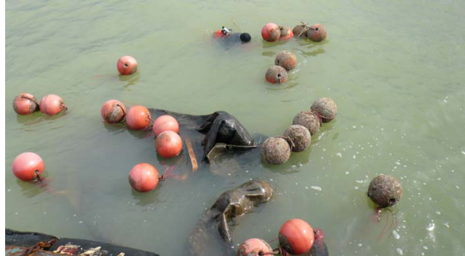
Recovering of A.R. silt curtain (1)
