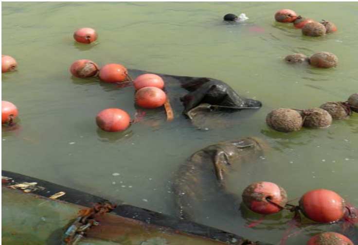
Recovering of A.R. silt curtain (2)
