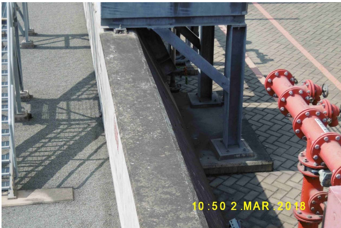
(16) This shows the thickness of the bund wall provided
