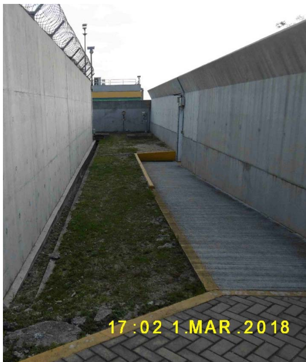
(10) Two impervious security walls are provided outside the bunded compounds
