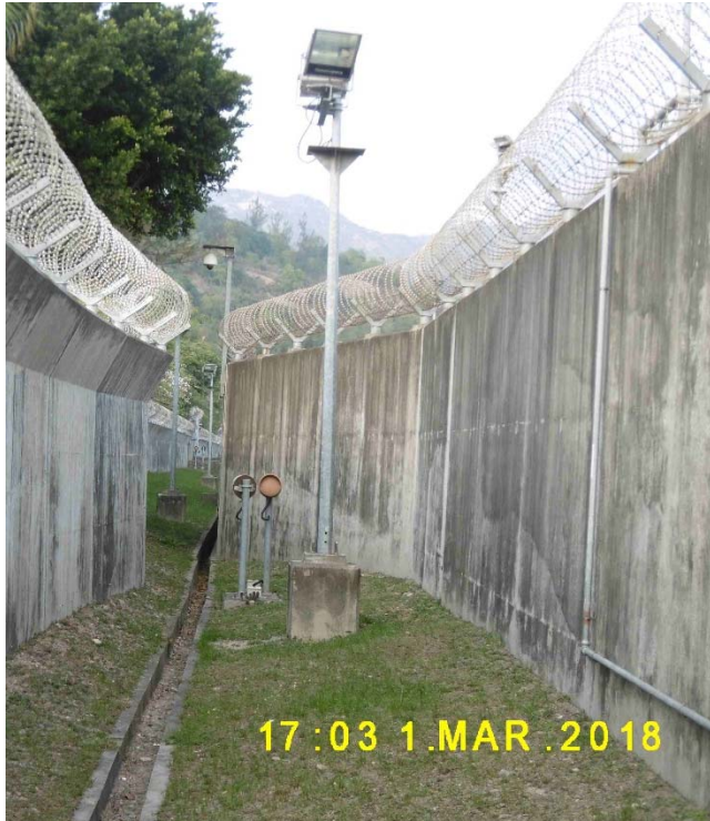
(11) Two impervious security walls are provided outside the bunded compounds
