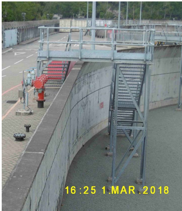
(5) Wave deflector are installed at top of the bunds
