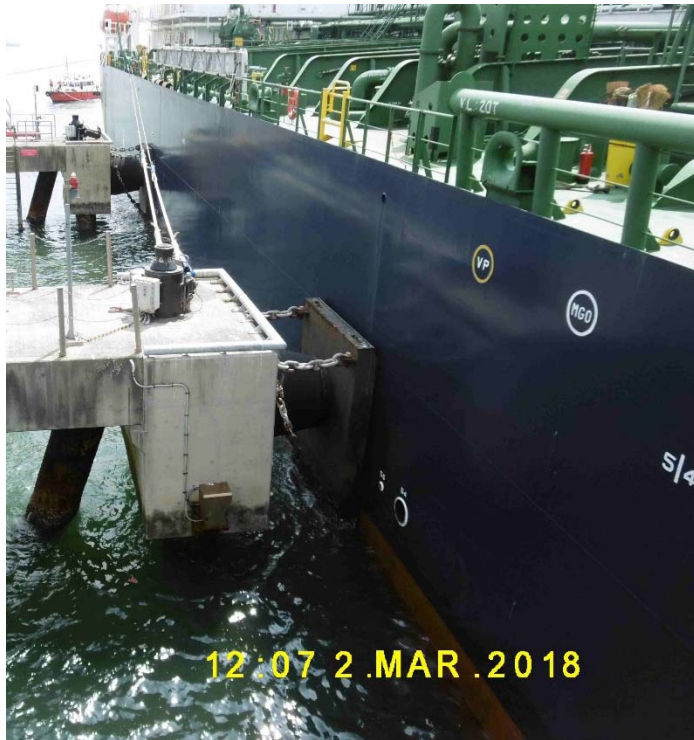
(37) Fenders are installed at sea side of the jetty
