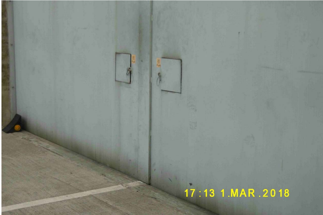
(15) Gates at security walls with sealant are maintained in good condition
