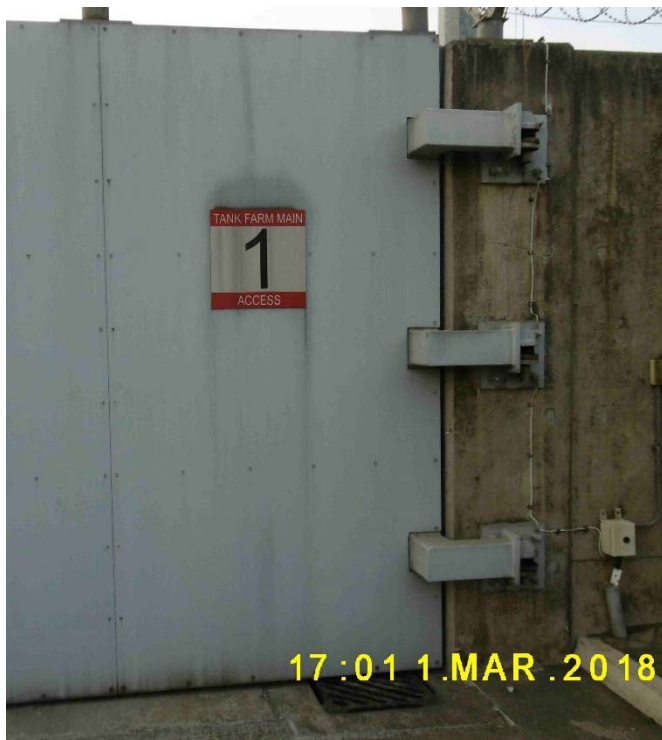
(14) Gates at security walls with sealant are maintained in good condition
