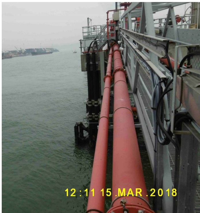
(38) Fenders are installed at shore side of the jetty
