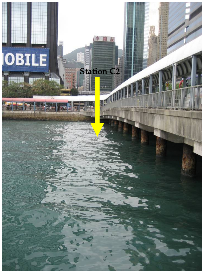
Additional Water Quality Monitoring Location – Station C2
