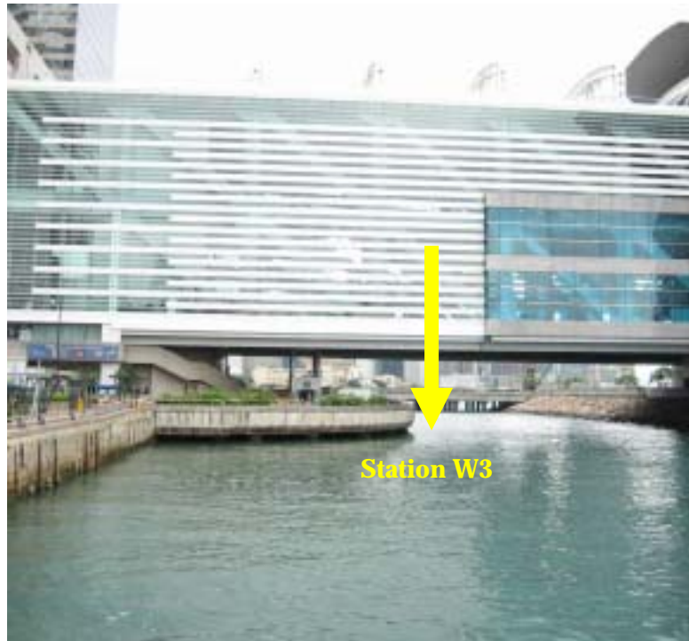
Water Quality Monitoring Location – Station W3
