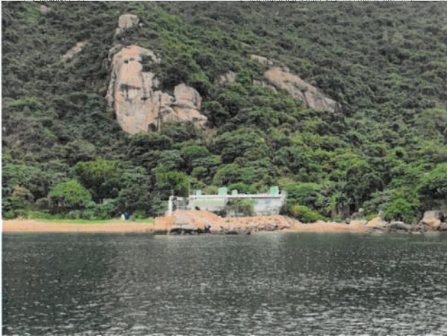
14 June 2022 Flood Tide (No construction activities)
