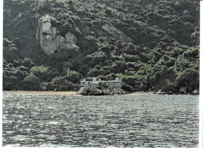
14 March 2023 Ebb Tide (No construction activities)
