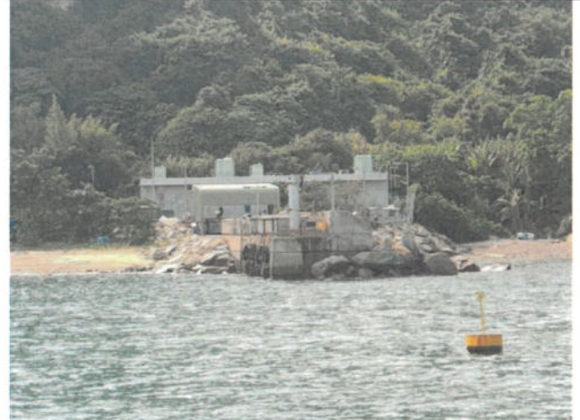
7 December 2022 Ebb Tide (No construction activities)
