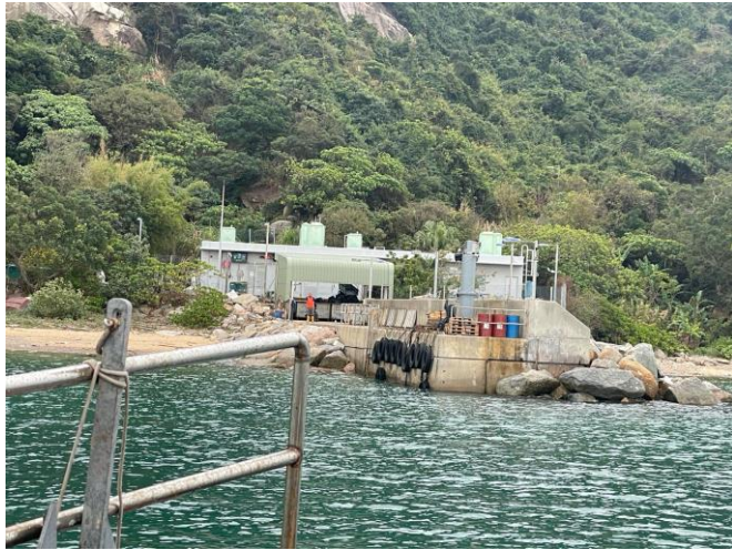
2 March 2024 Flood Tide (No construction activities)
