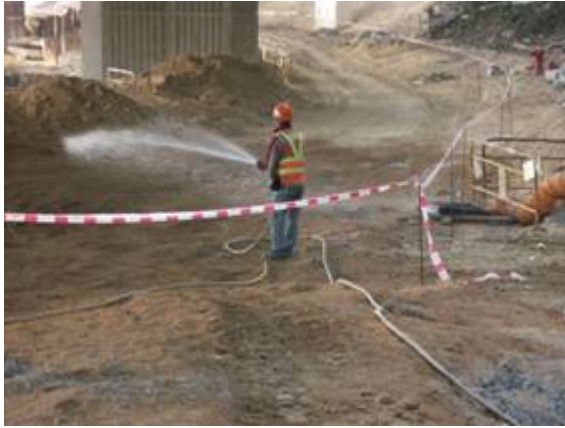
Photo 01 (area P2-SA6B (under the bridge C2/D2))
