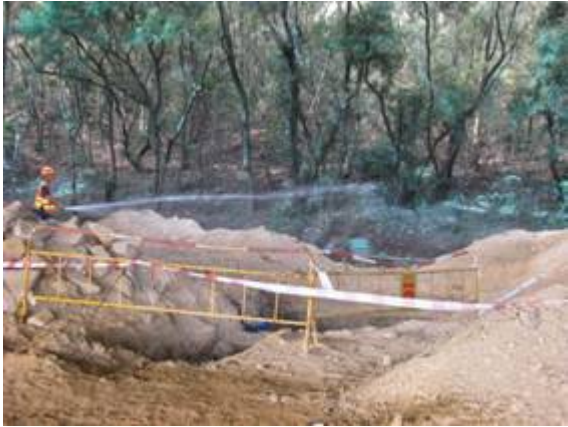
Photo 08 (area P2-SA6B (under C2/D2 Bridge))
