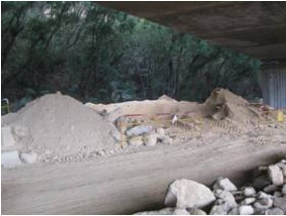
Photo 07 (area P2-SA6B (under C2/D2 Bridge))
