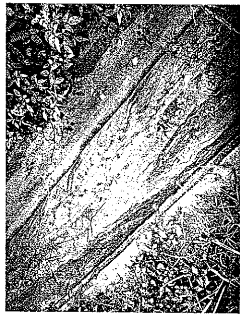
Photo 110125_004 (Drainage channel near chemical waste storage area)
