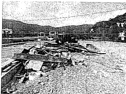
Fig.11 – Site clearance to be carried out at PNH maintenance ramp
