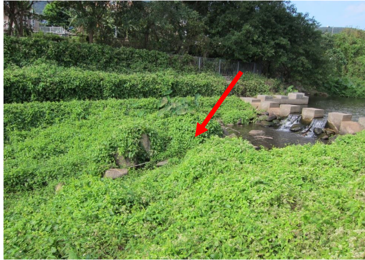
Mile-a-minute partially blocks the water flow at the fish ladder
