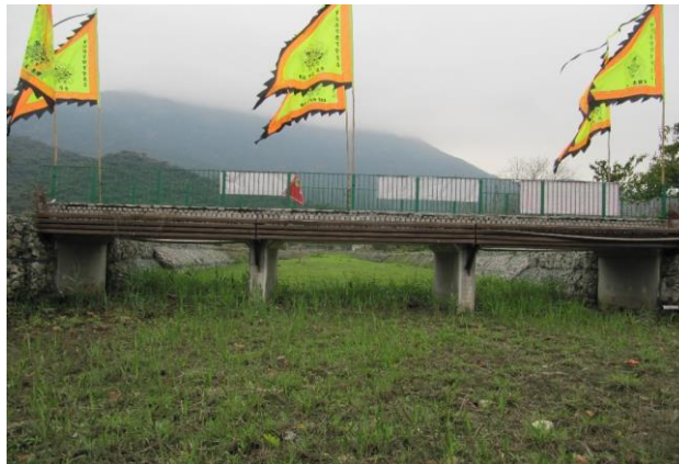
Re-establishment of vegetation along LBC
