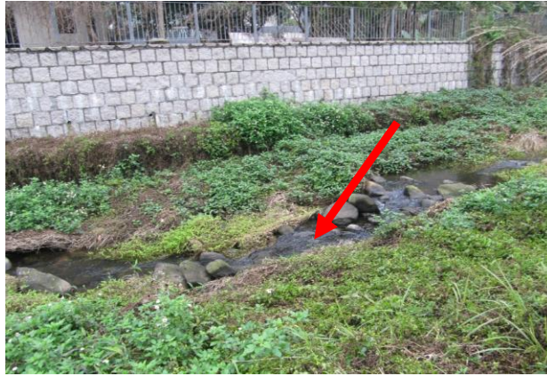
Vegetation was overgrown, but water can still freely flow along the fish ladder
