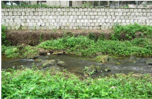
Condition of the fish ladder in PNH3 and PNH4
