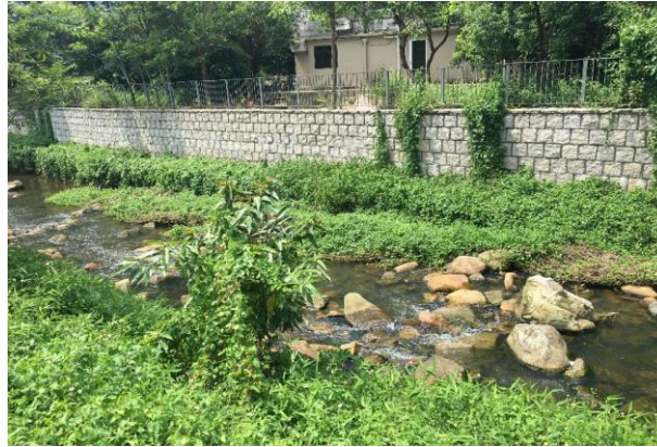
Condition of the fish ladder in PNH3 and PNH4
