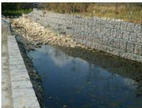
Fig.3 – Condition of PNHR, fish ladder section
