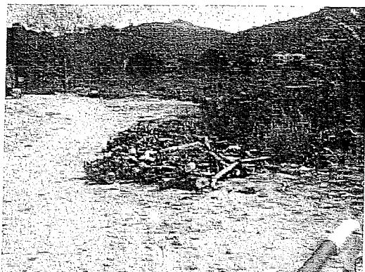
Fig.13 – Site clearance to be carried out at TTTR bottleneck A
