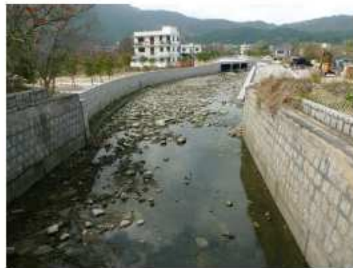
Fig.2 – Condition of PNHR (downstream area)
