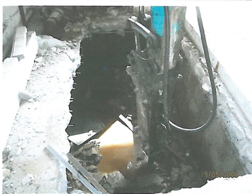
Trial pit no. GFSA-06 inside the Generator Room
