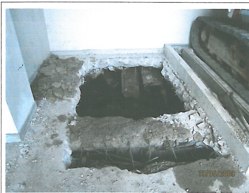
Trial pit no. GFSA-07 inside the Generator Room
