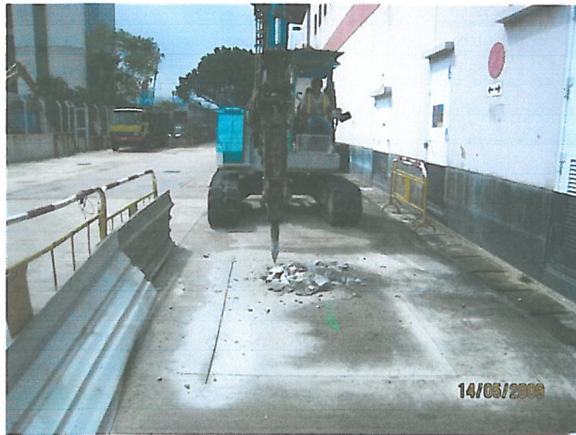
General view of relocated trial pit no. GFSA-05
