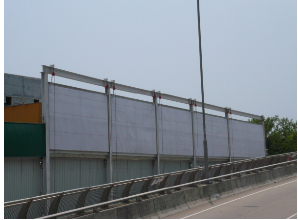
Photo 13: Noise barrier along Cyberport Road
