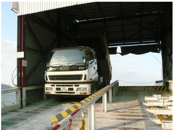
Photo 7: Dump truck discharging excavated materials onto the barge at the ramp jetty
