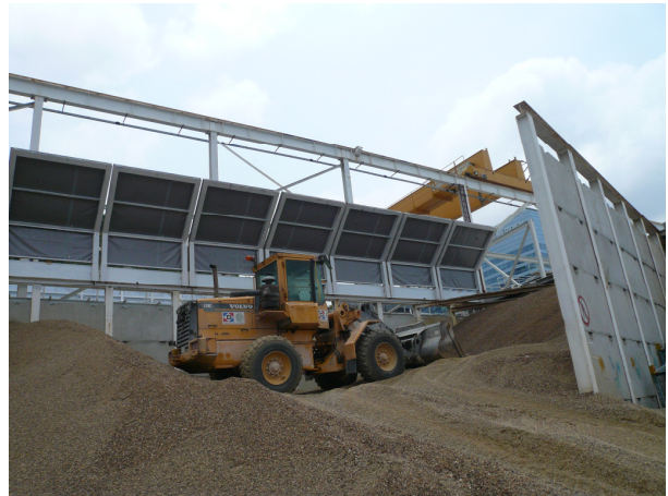
Photo 12: Noise barrier at the pea gravel storage yard at the side facing Aegean Terrace
