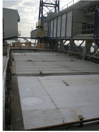
Photo 11: Noise covers at the Adit Spoil Basin
