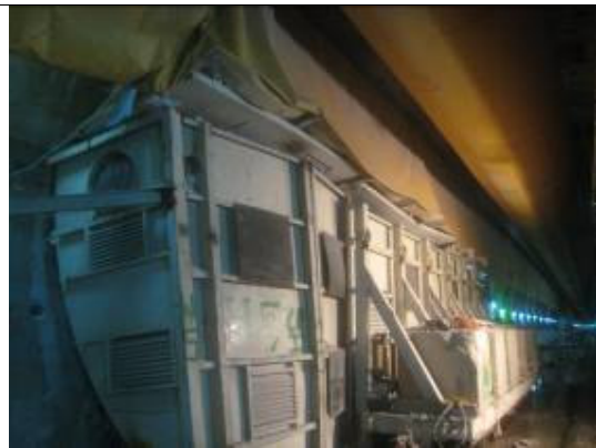
Blast door at tunnel and adit junction for micro-blasting
