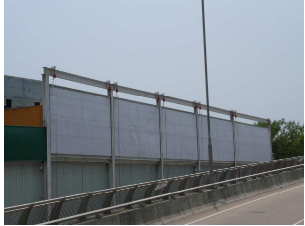
Photo 13: Noise barrier along Cyberport Road
