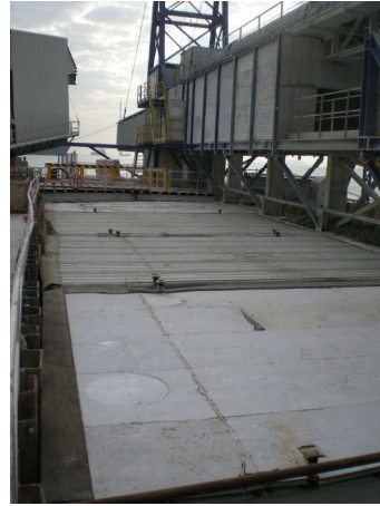
Photo 11: Noise covers at the Adit Spoil Basin
