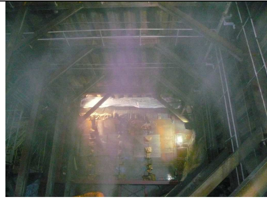
Water sprinkler system for dust & fumes suppression
