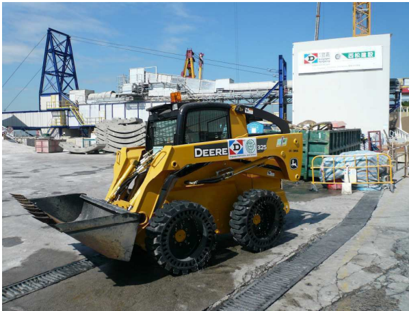
Photo 3: John Deere Skid Loader
