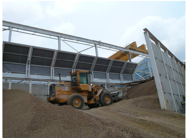
Photo 12: Noise barrier at the pea gravel storage yard at the side facing Aegean Terrace
