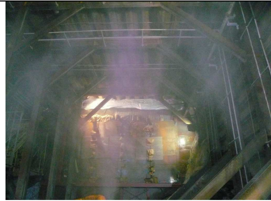
Water sprinkler system for dust & fumes suppression
