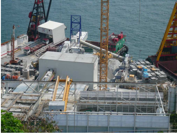
Photo 8: Covered Conveyors
