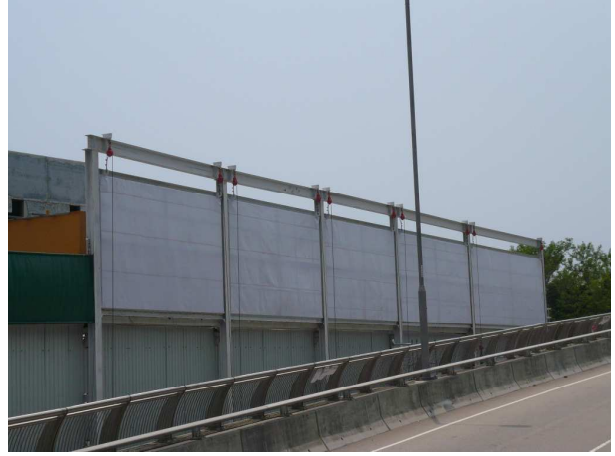
Photo 13: Noise barrier along Cyberport Road
