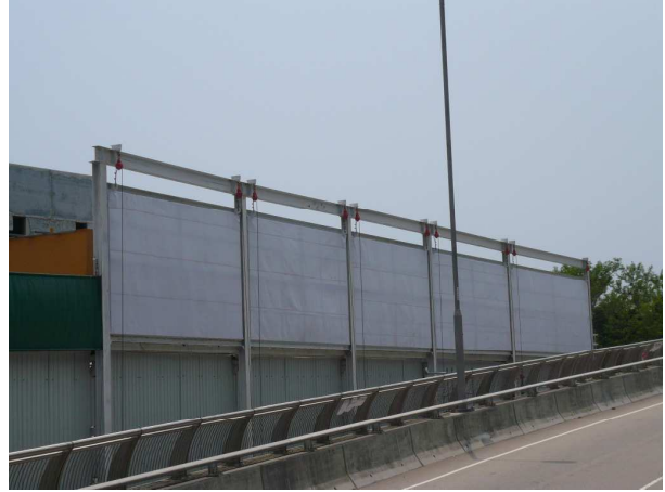
Photo 13: Noise barrier along Cyberport Road
