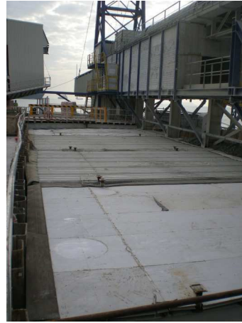
Photo 11: Noise covers at the Adit Spoil Basin
