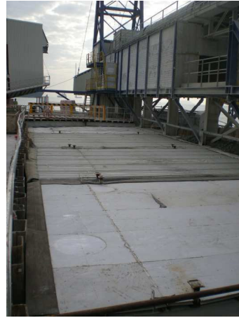
Photo 11: Noise covers at the Adit Spoil Basin
