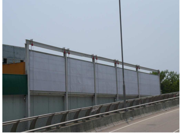
Photo 13: Noise barrier along Cyberport Road
